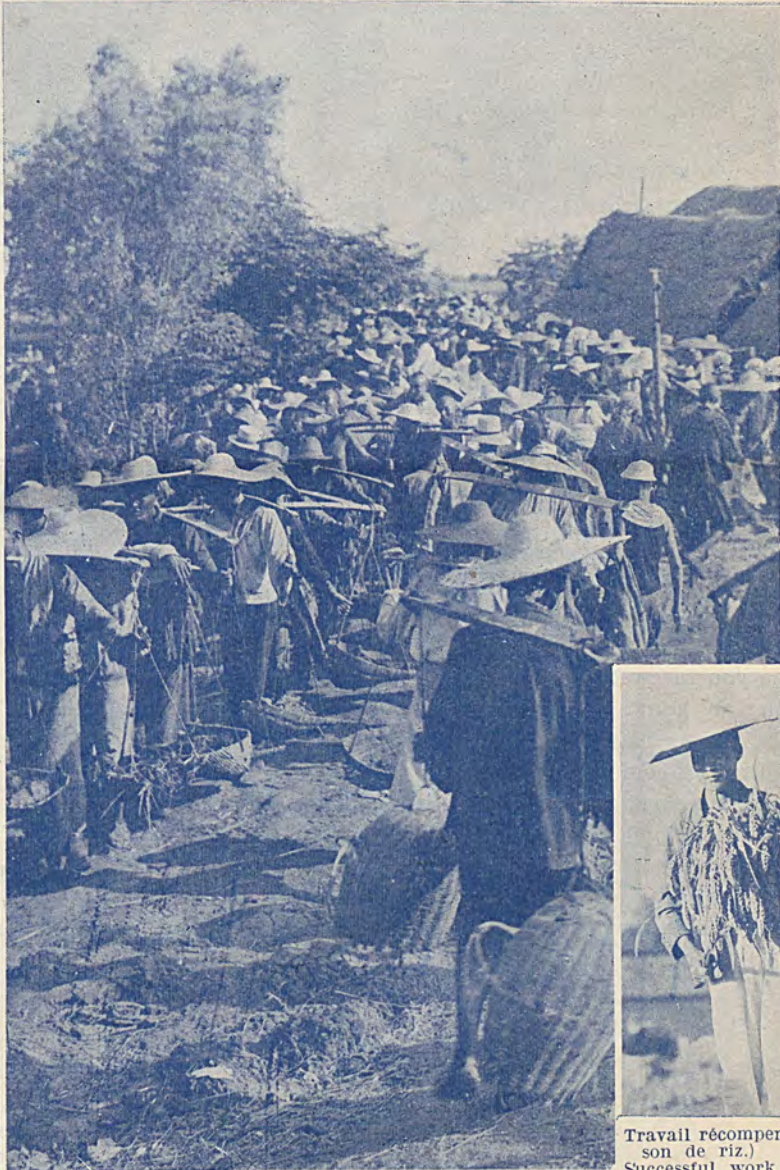
Terrassements. Earth-works. Dammarbeiten
